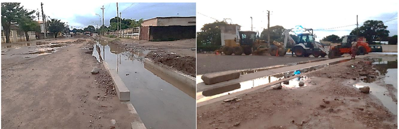
Fig. 6. Drainage being built along roads at Machava-Sede (photos: author).
