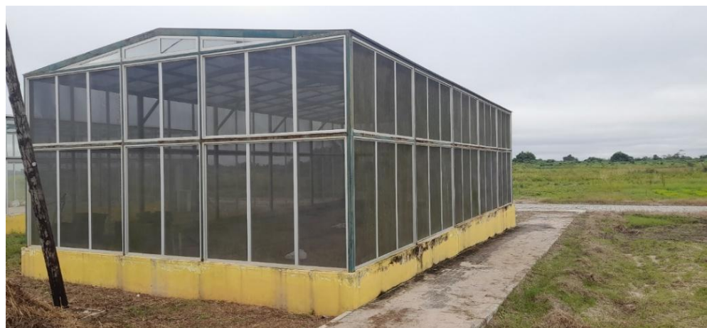
Figure S1.1. Greenhouse where the study was conducted (Length = 15 m; Width = 8 m; Height = 4.2 m). Walls made of iron mesh and aluminum and iron poles, with glass roof. Location GPS: 17°29'35.1" S, 37°00'34.0" E.
