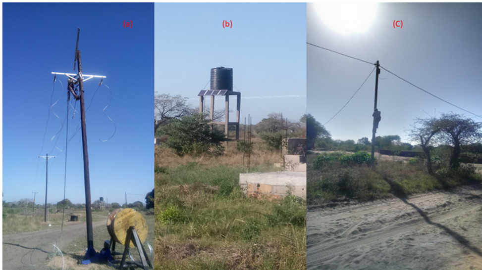
Figure 7. Examples of electrification of rural areas in Mozambique using on-grid system in (a) and (c) by EDM and using an off-grid PV system for water supply by FUNAE (b) (photo by Miguel M. Uamusse).
